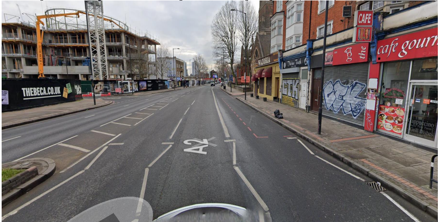
View looking south-east along Old Kent Road showing residential dwellings being built opposite the premises
